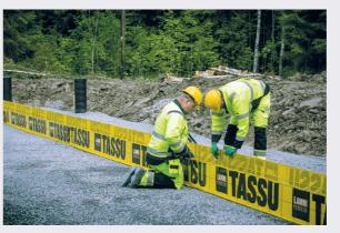
Ready-made molds are installed on a levelled and firm ground.
