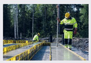
After installing any additional reinforcements, the ready-made mold is cast with concrete and the upper surface is levelled at the correct height.
