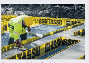
Once the concrete is dry, there is no need to dismantle the mold. This way the plot remains free of construction waste.
